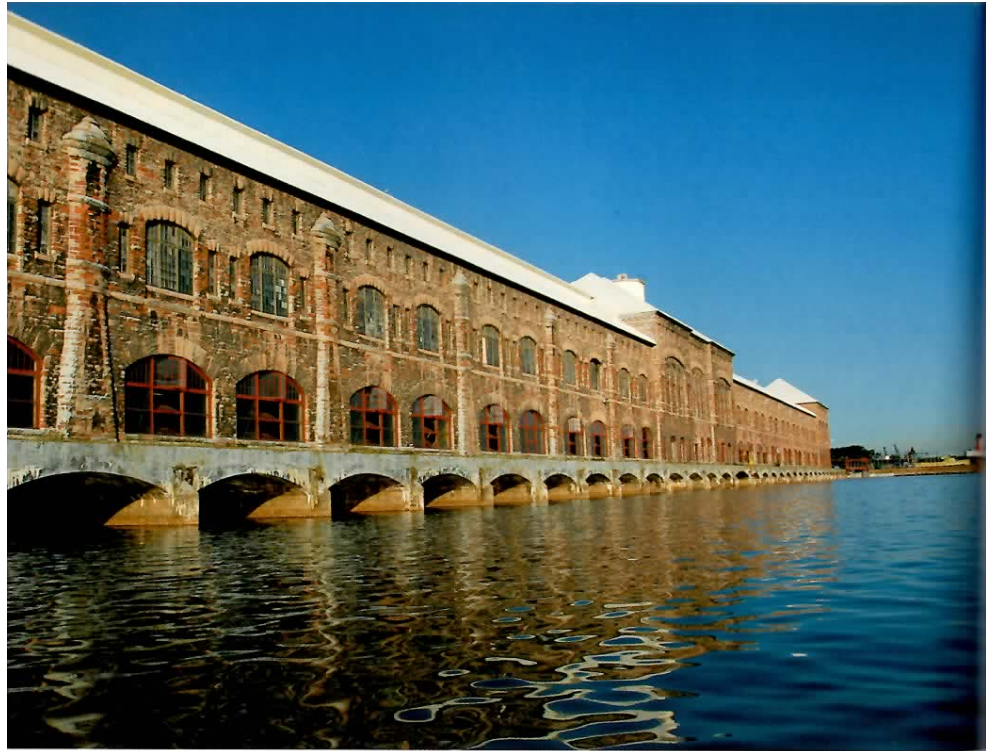
is a building where electricity is created from the river water passing underneath it. Shooting from a boat, I used the long horizontal lines and a wide depth of field to make the building seem to stretch out into the distance.
